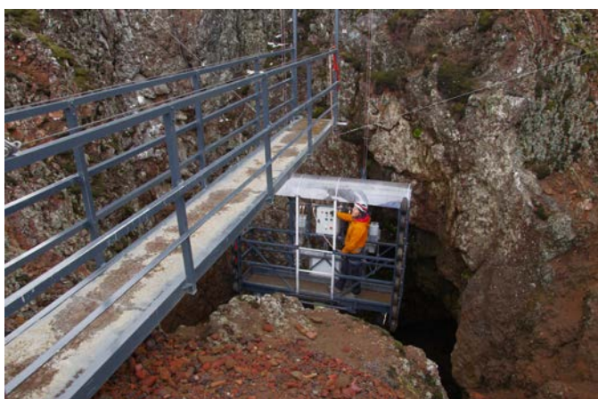
View of the approach walkway and lift platform for the Inside The Volcano descent. The wheels on the side of the platform are to keep it clear of the walls in a narrow part of the shaft. Photo: John Brush
